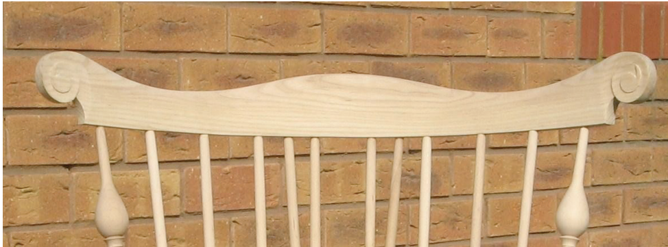
The steamed and bent crest piece in American white ash.
