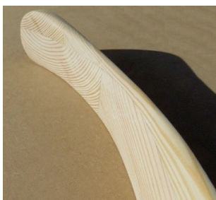
Photo 4-78p. Overhead view of the end of the completed crest showing the curved top and the splayed face.
